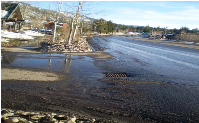
Photo 1.1. Directly Connected Drop Inlet to Burke Creek
