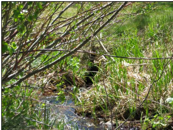
May 9, 2012. WOUS 1, Burke Creek. View downstream (southwest) of US50 east side culvert.
