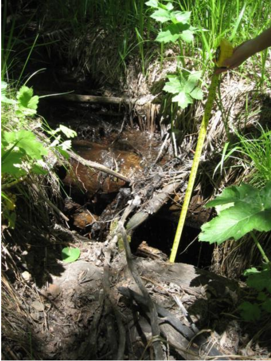
3' deep headcut on the north channel split.
