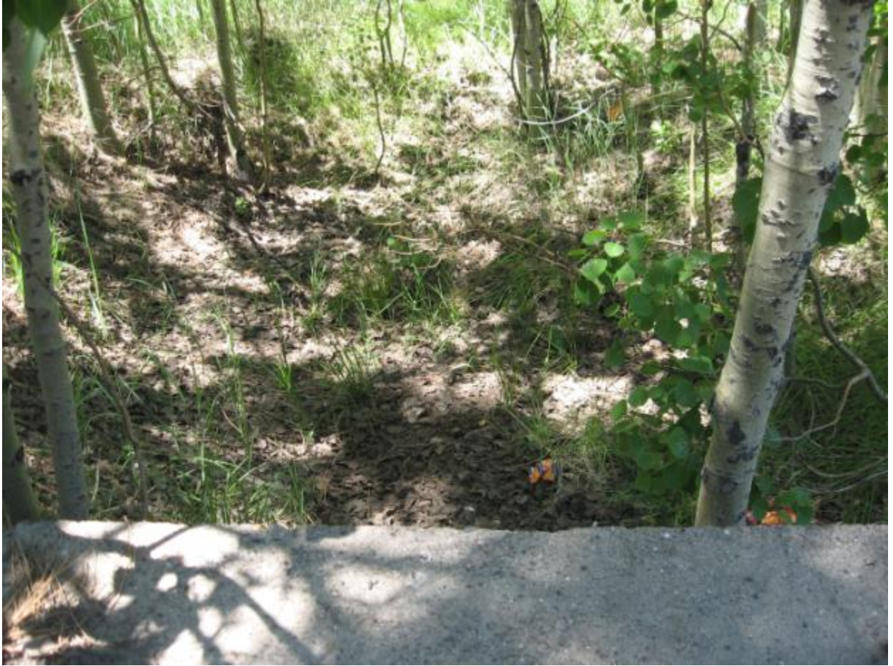
The small natural basin at the discharge point DCDP0087 of HWY 50 culvert crossing DCCP0466.
