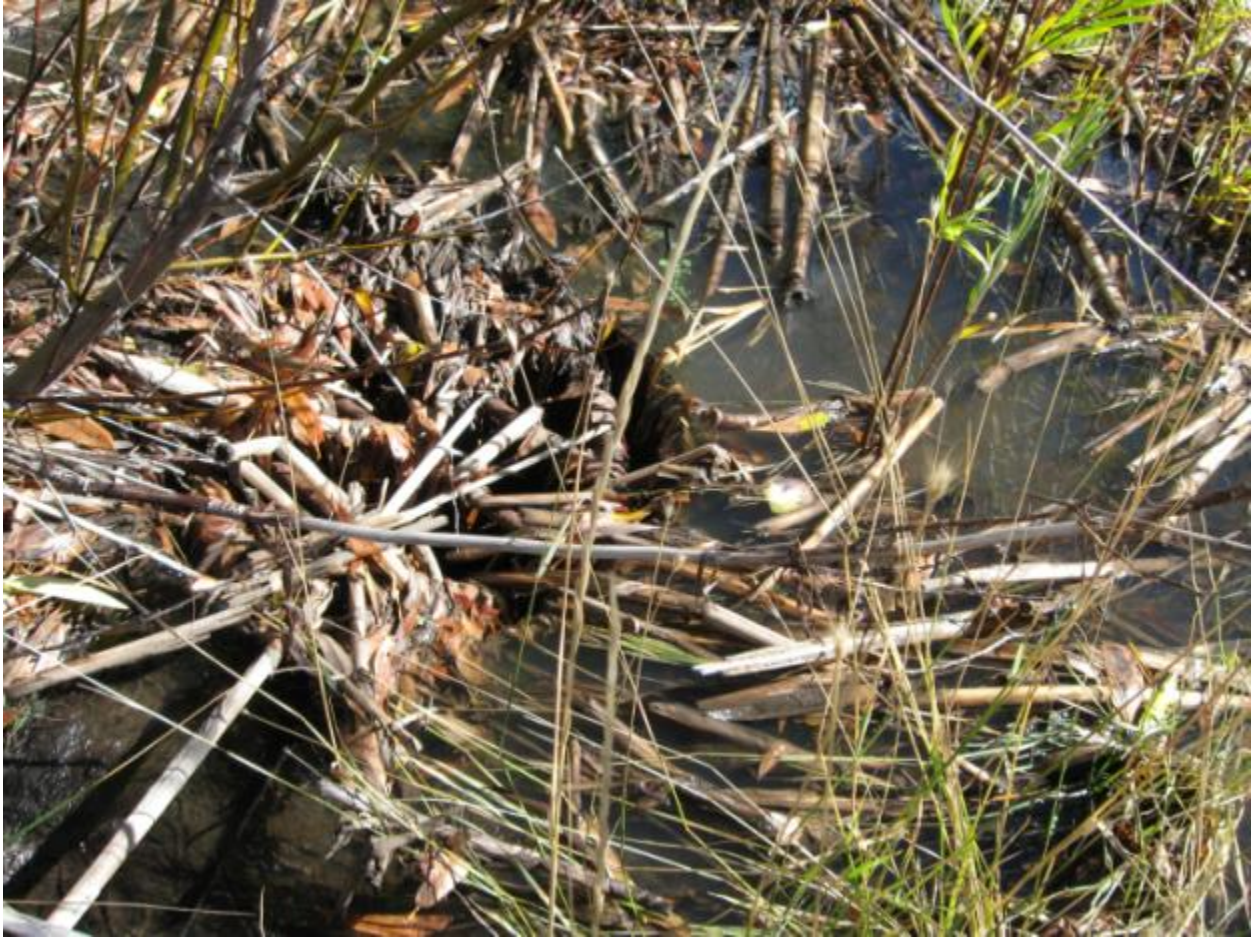
Kahle Basin standpipe DCDO0025 with no sump. Basin had 18" sump when constructed.
