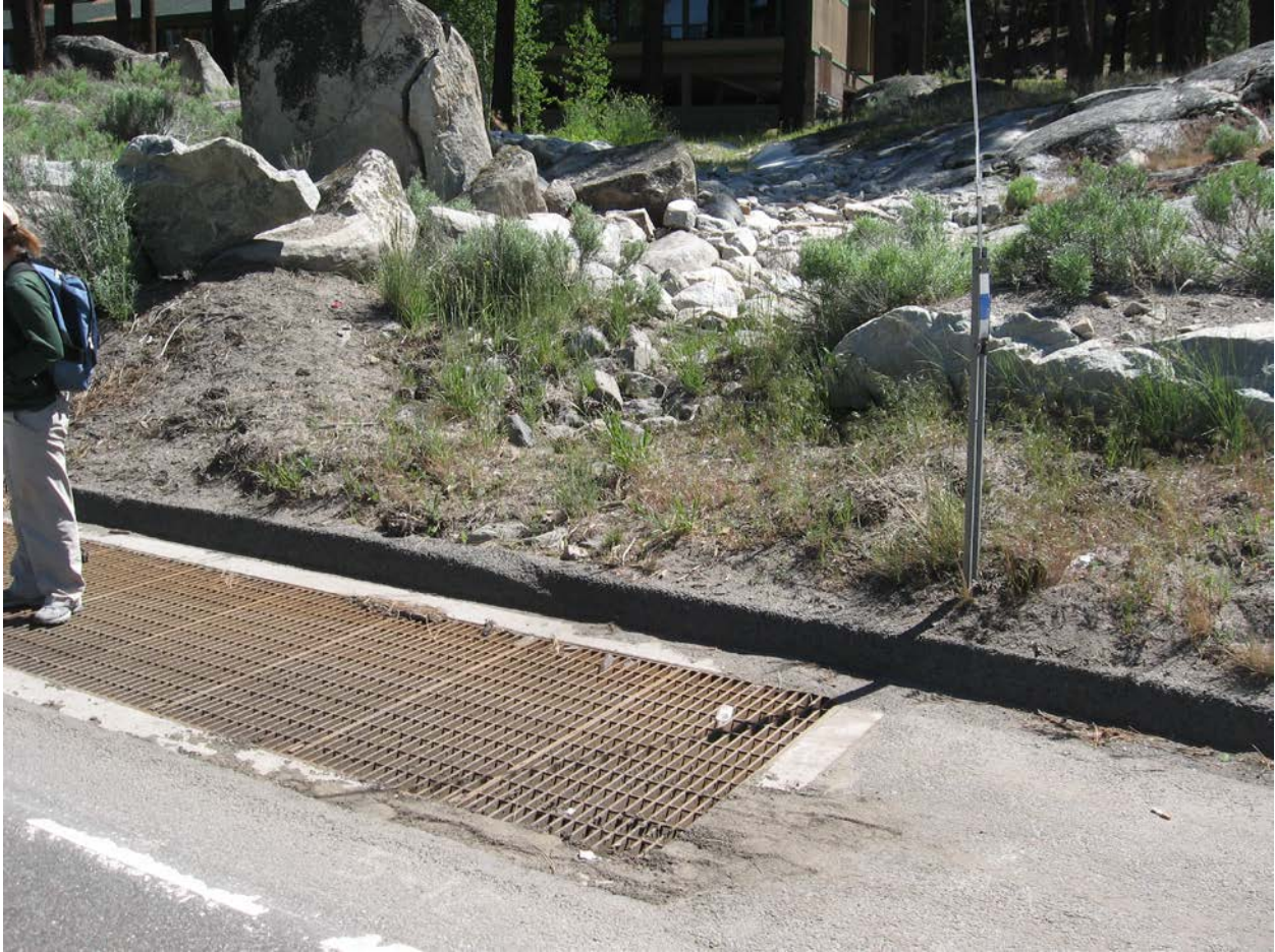
Lake Village Phase II outfall from rock-lined swale to NDOT trench drain DCCD0168.
