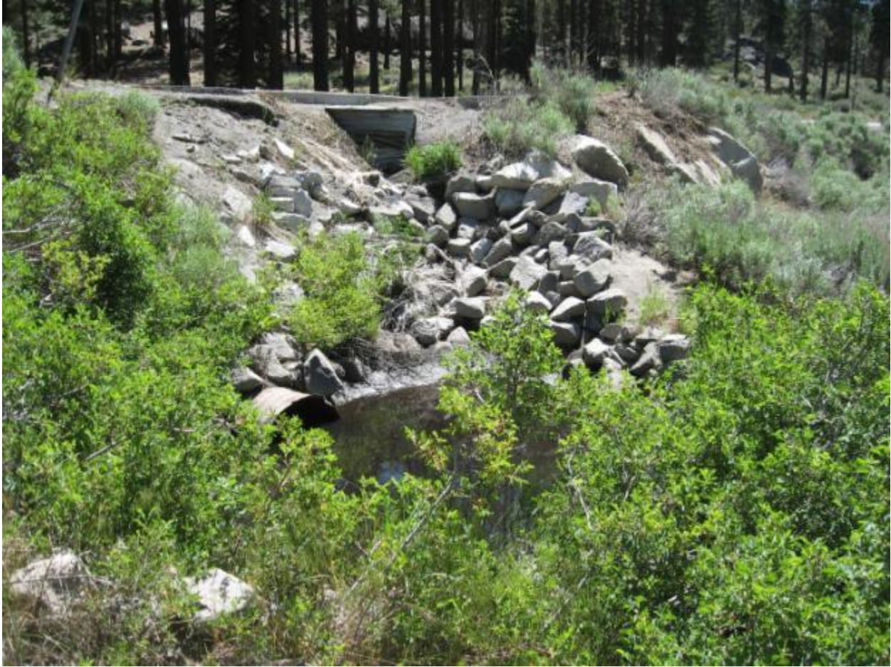
Discharge point of rock-lined channel DCCD0166 and culvert DCCP0458 from HWY 50 culvert crossing.
