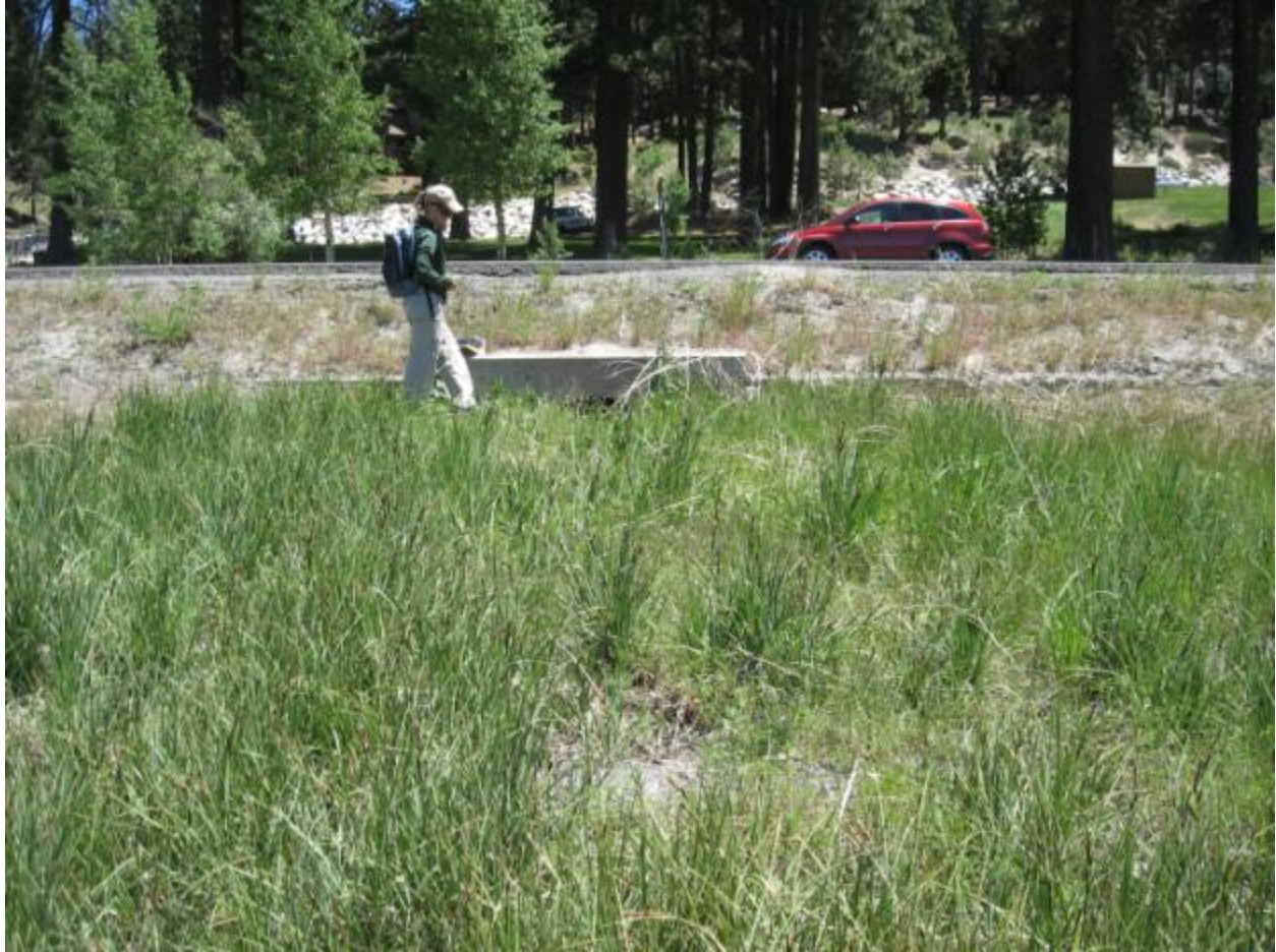
Outfall DCOF0044 of HWY 50 culvert crossing DCCP0465 and rip rap dissipater DCBS0138.
