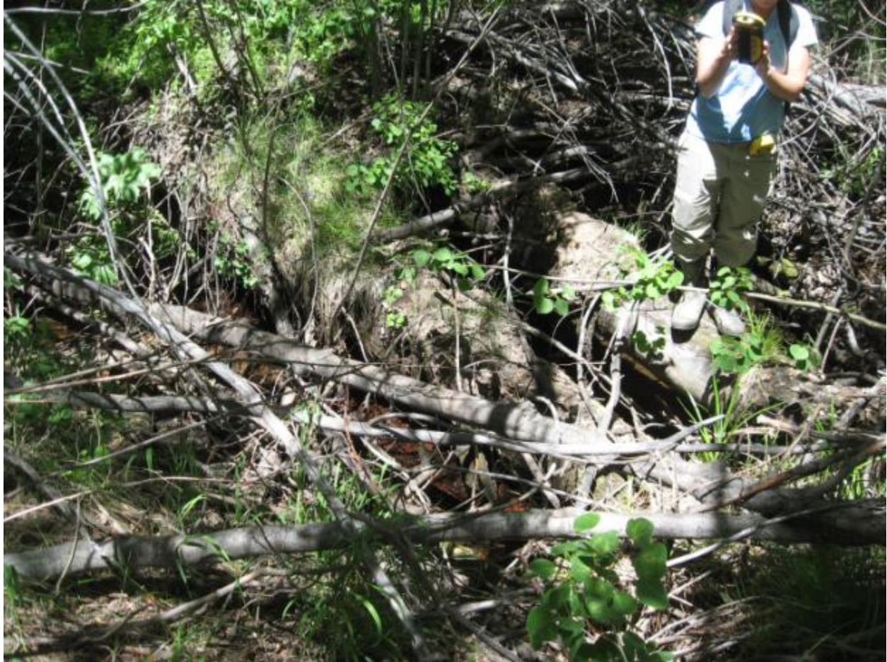
Channel split and upper end of headcuts (2 headcuts –1 on each split channel). Logs pictured were once buried and are now exposed due to creek undercutting.
