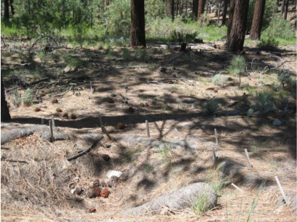
Spreading area of culvert DCCP0457 discharge point from HWY 50 crossing.
