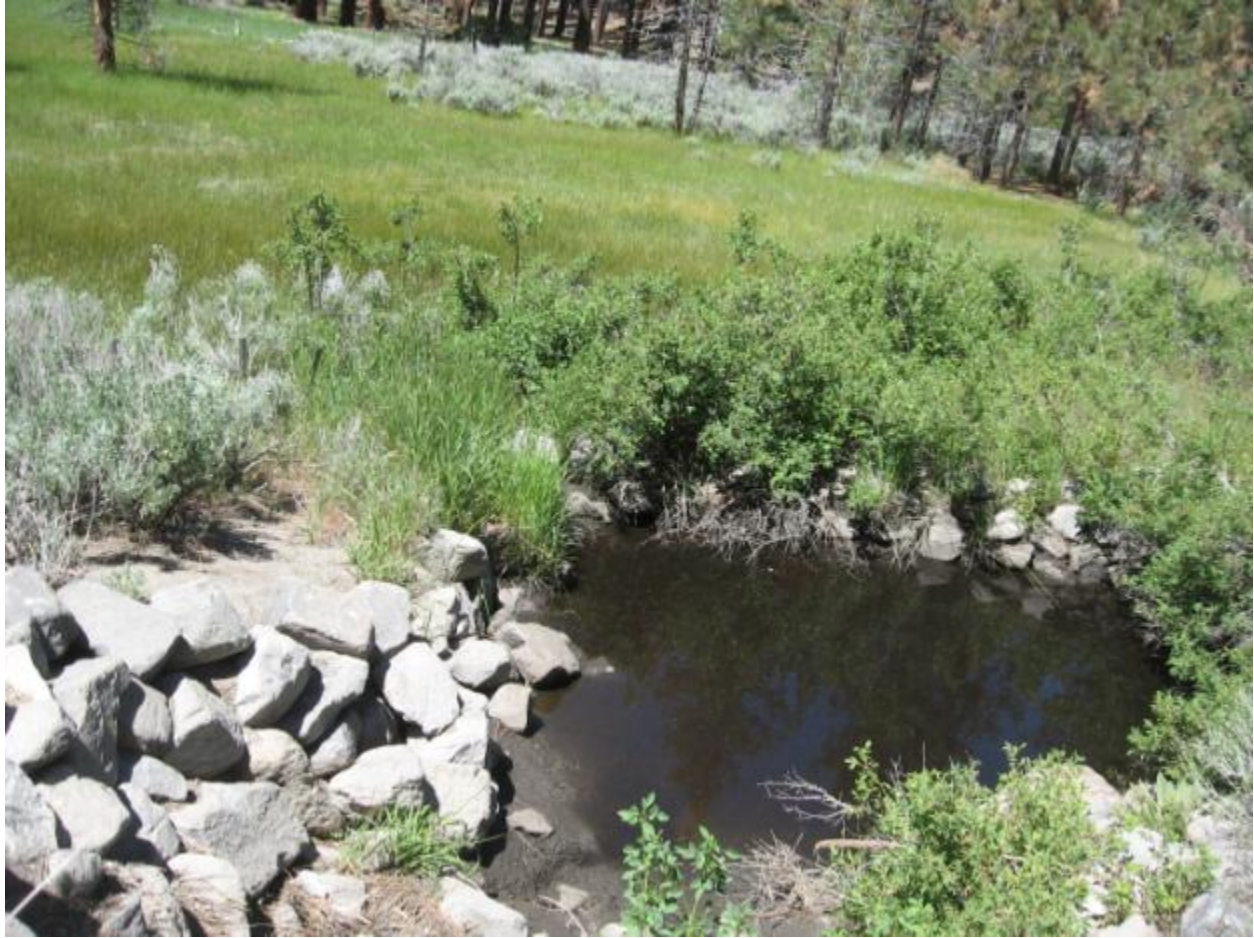
Spreading area of Rip Rap dissipater DCBS0191.
