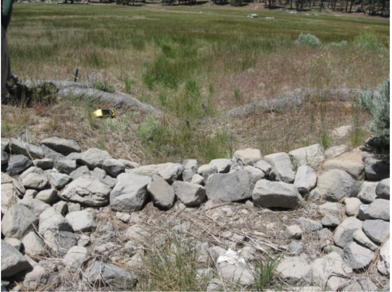
Spreading area of rip rap dissipater DCBS0136 and discharge point of HWY 50 crossing culvert DCCP0463.
