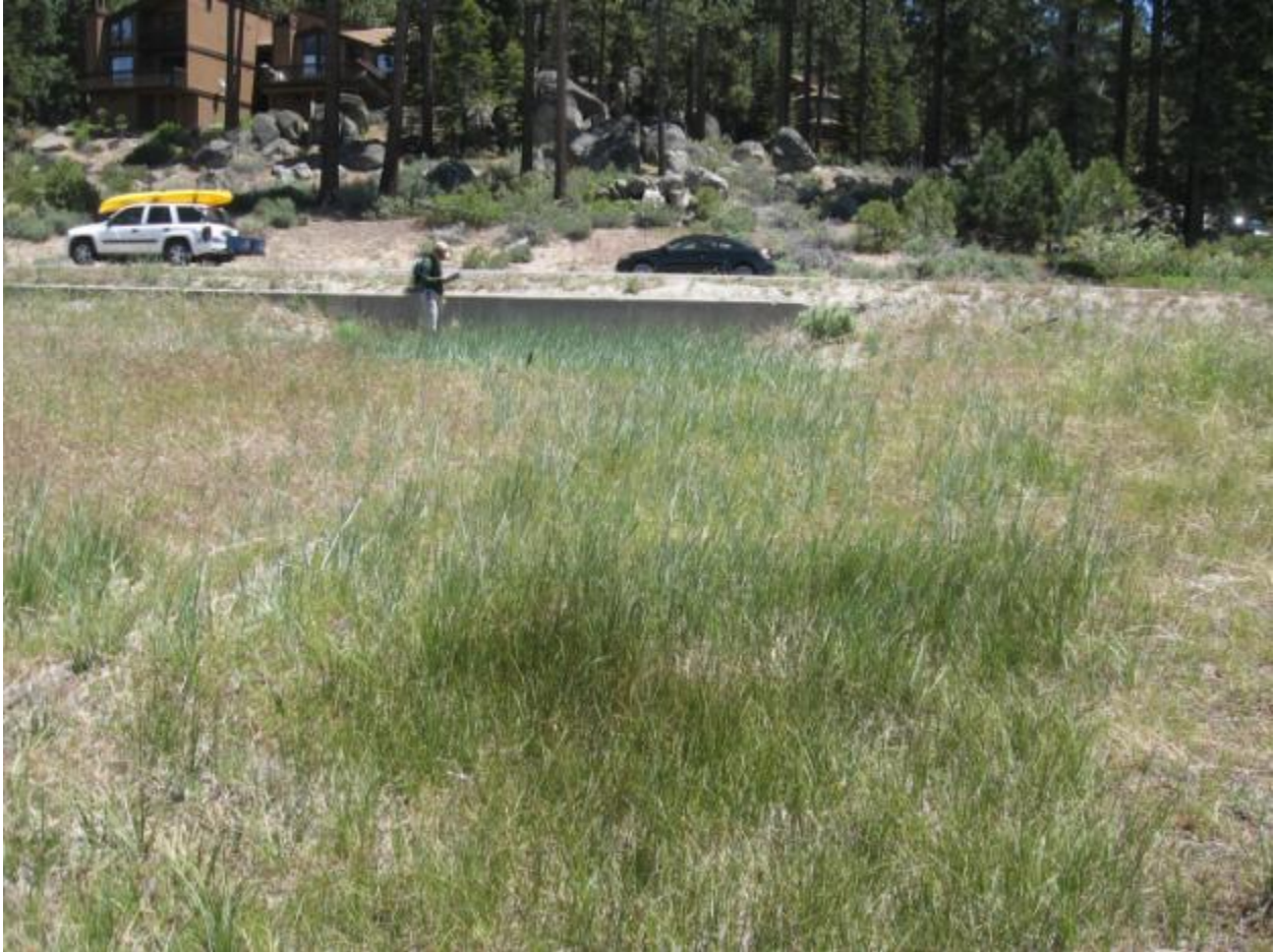
Outfall DCOF0074 of HWY 50 culvert crossing DCCP0464 and rip rap dissipater DCBS0137.
