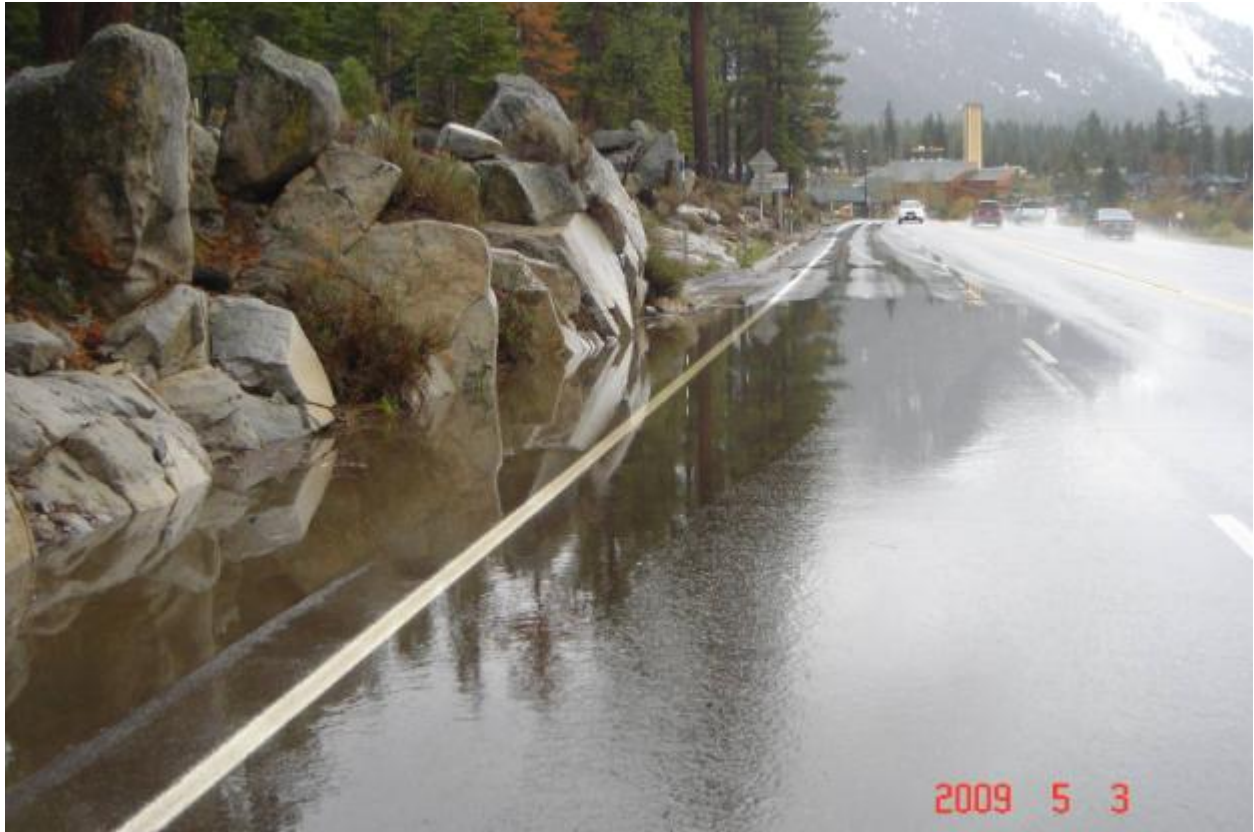
Hwy 50 flooding of eastbound lanes #1 and 2.
