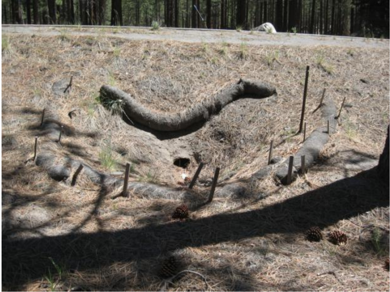
Discharge point of culvert DCCP0457 from HWY 50 culvert crossing.
