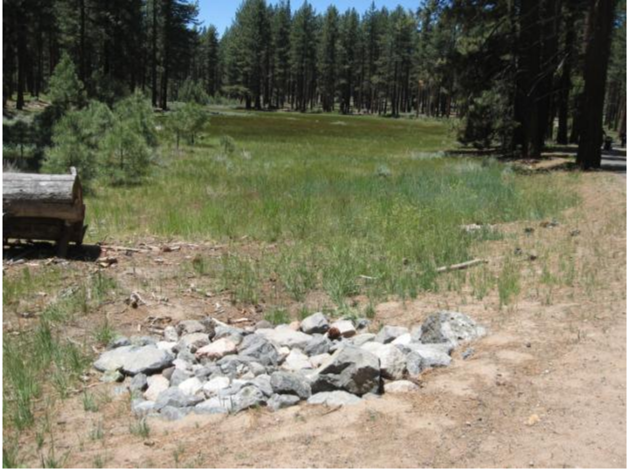
Spreading area of rip rap dissipater discharge point of Stateline to Stateline bike path culvert.
