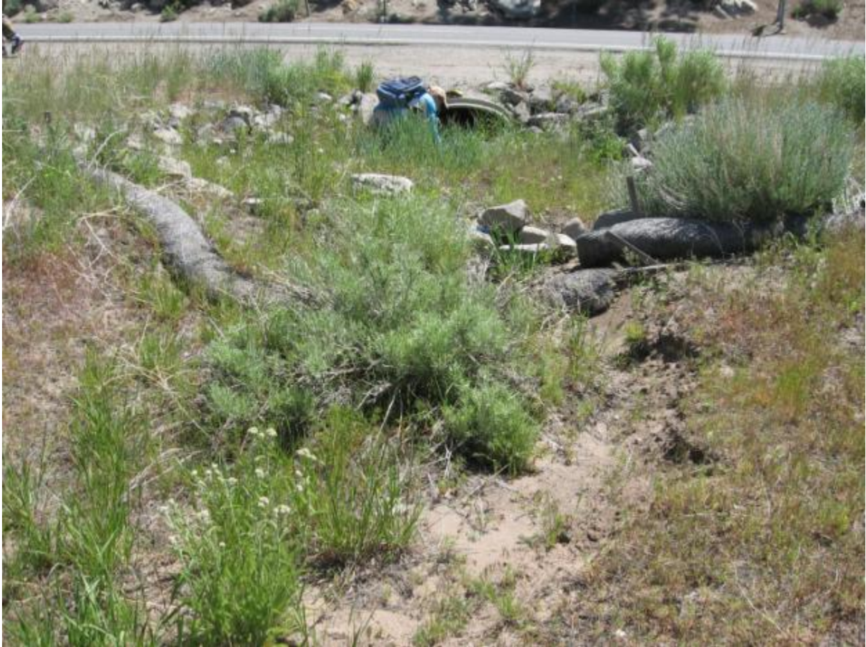
Discharge Point DCDP0088 of HWY 50 culvert crossing DCCP0469. The runoff is discharged to private property.
