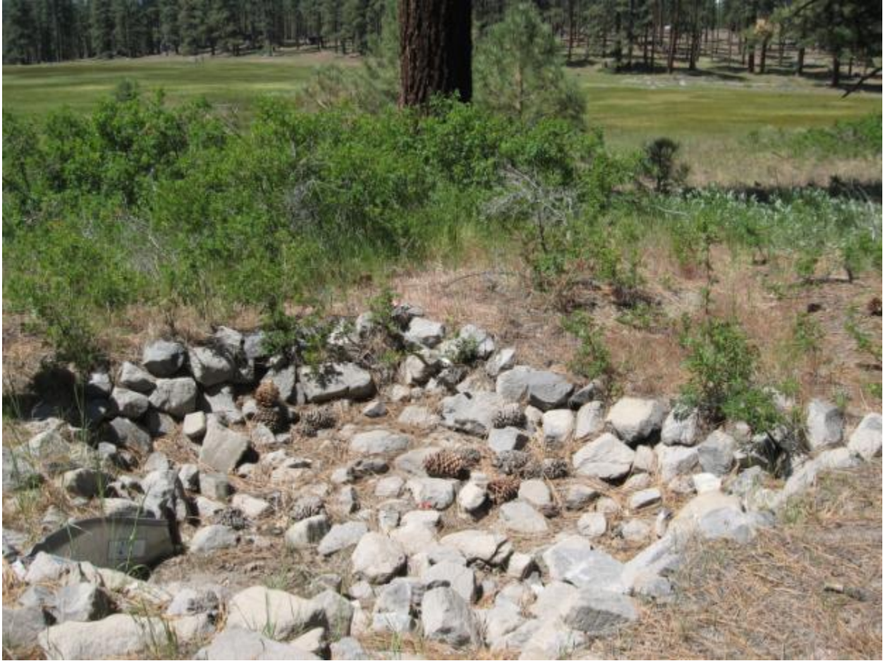
Spreading area of rip rap dissipater DCBS0134 and discharge point of HWY 50 crossing culvert DCCP0460.
