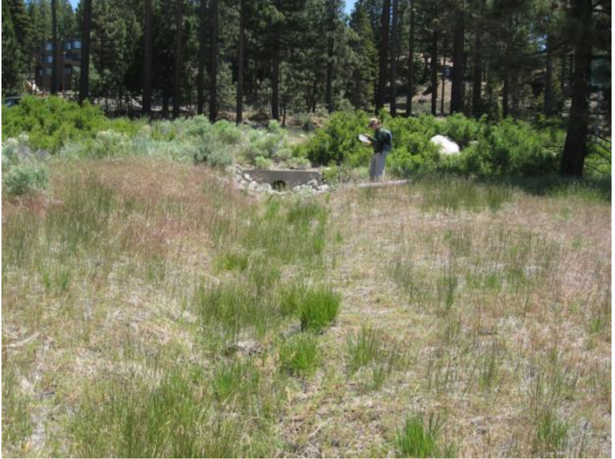
Discharge point of HWY 50 culvert crossing DCCP0463 and rip rap dissipater DCBS0136.
