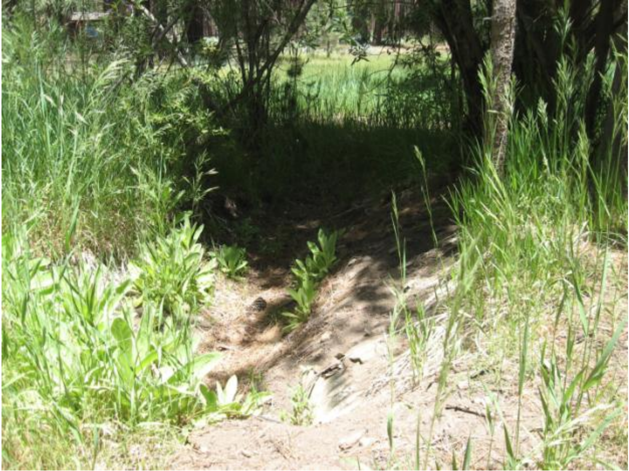
Looking upstream at meadow drainage from the culvert crossing the Nevada Beach campground road. 18" aluminum culvert. 6' wide x 18" deep channel. Pine needle/veg substrate.
