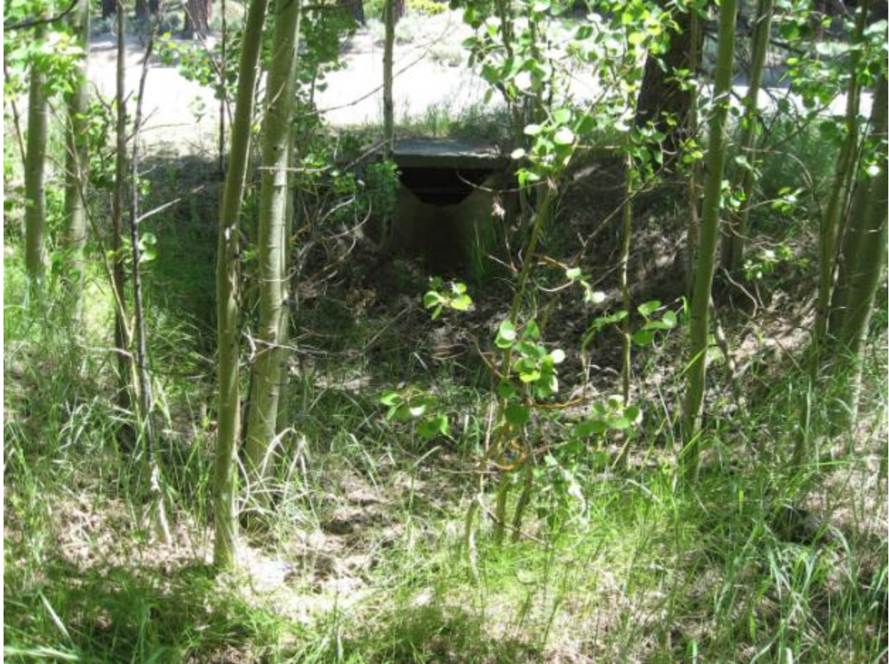
Discharge Point DCDP0087 of HWY 50 culvert crossing DCCP0466. A small natural basin exists at the discharge point.
