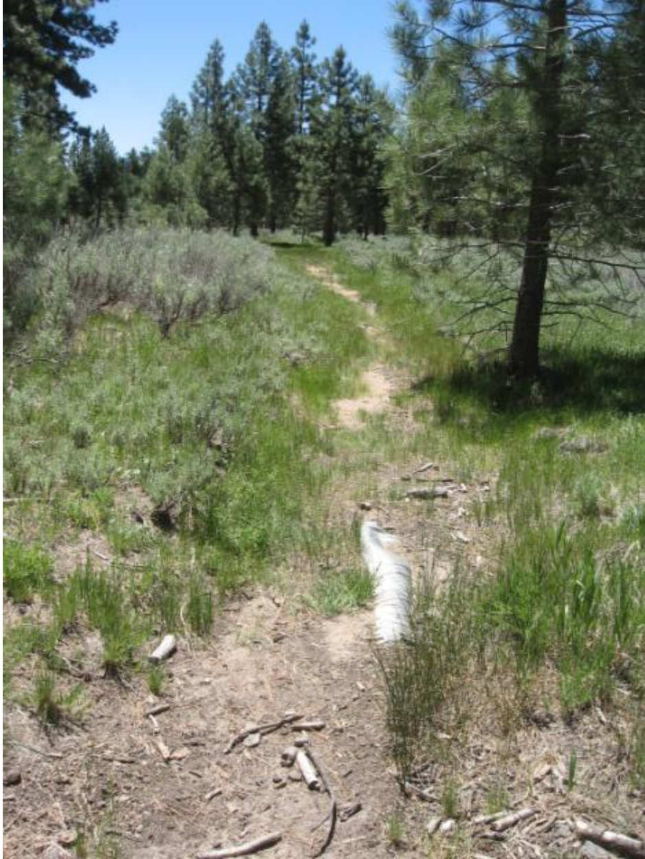
Flow path of drainage from culvert crossing use trail at north end of Rabe Meadow toward Nevada Beach. 6' wide x 8" deep channel. Vegetation/sand substrate. 2 rock weirs installed in channel to hold grade.
