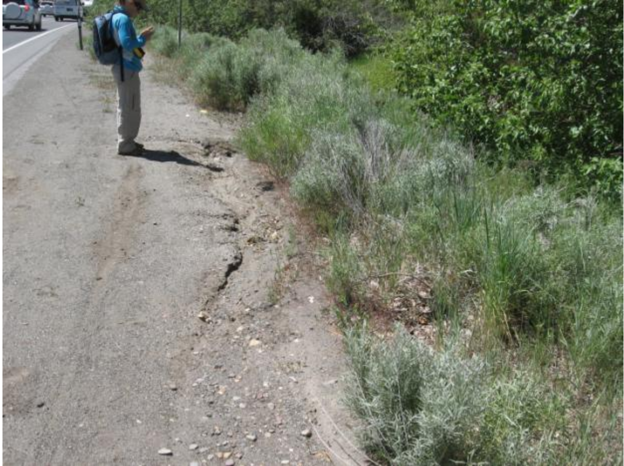
Eroded flow path from concentrated runoff along HWY 50 near Burke Creek. The runoff discharges to a use trail and eventually Kahle Ditch.
