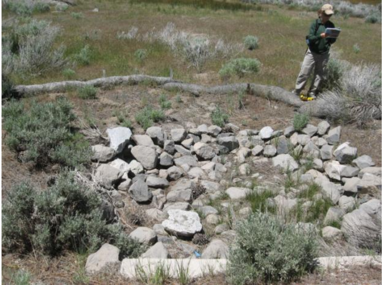
Spreading area of rip rap dissipater DCBS0135 and discharge point of HWY 50 crossing culvert DCCP0462.
