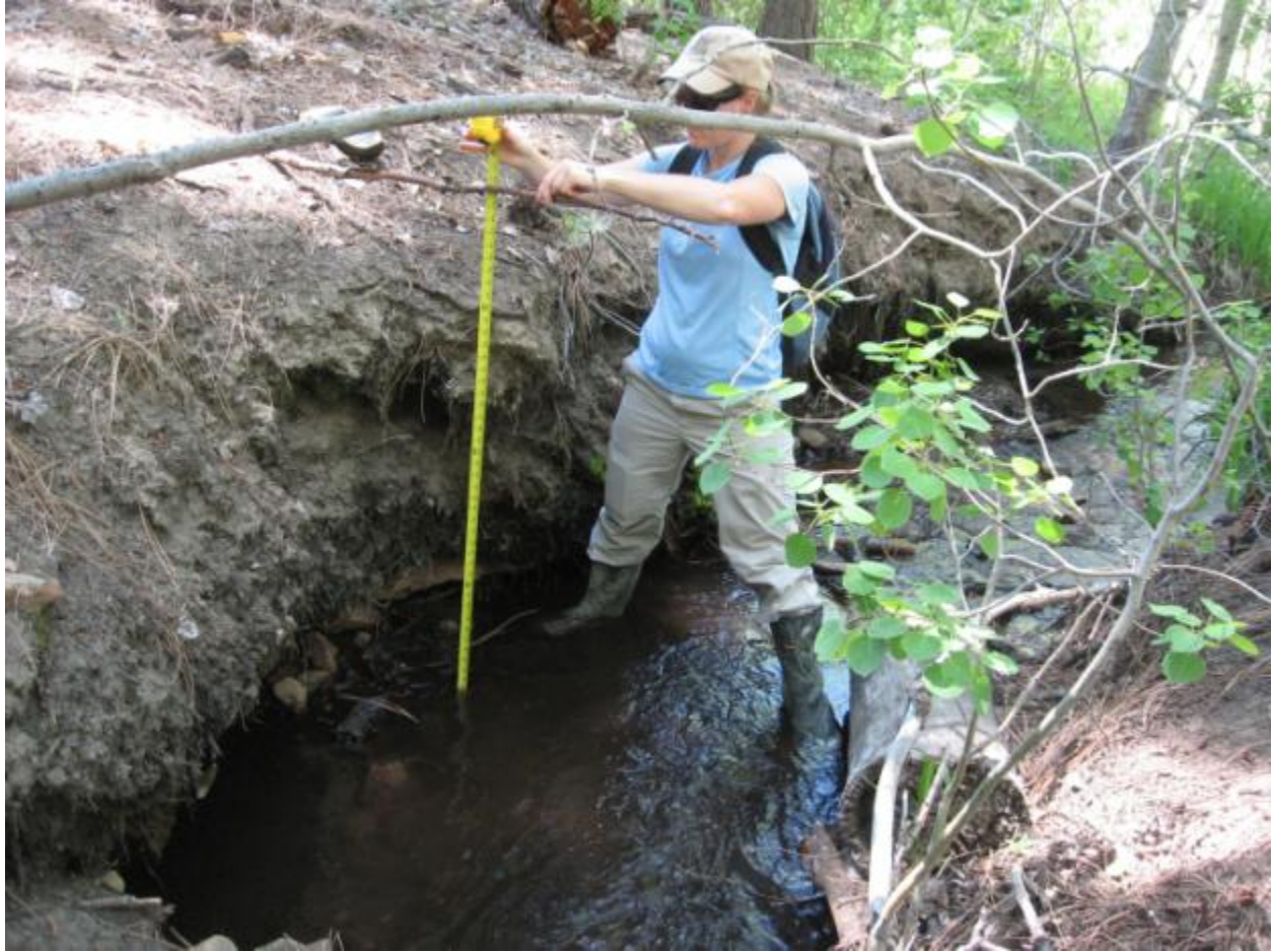
Eroded and undercut banks. Burke Creek has cut banks 3' deep.
