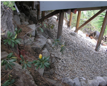
Figure 14: Armor under elevated
