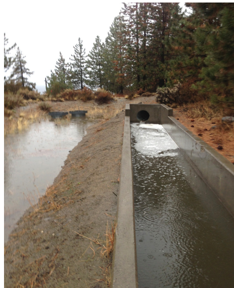
Figure 2: CRE Stormwater System 2011
