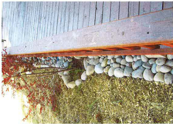
Erosion Control at Perimeter of Low Deck
