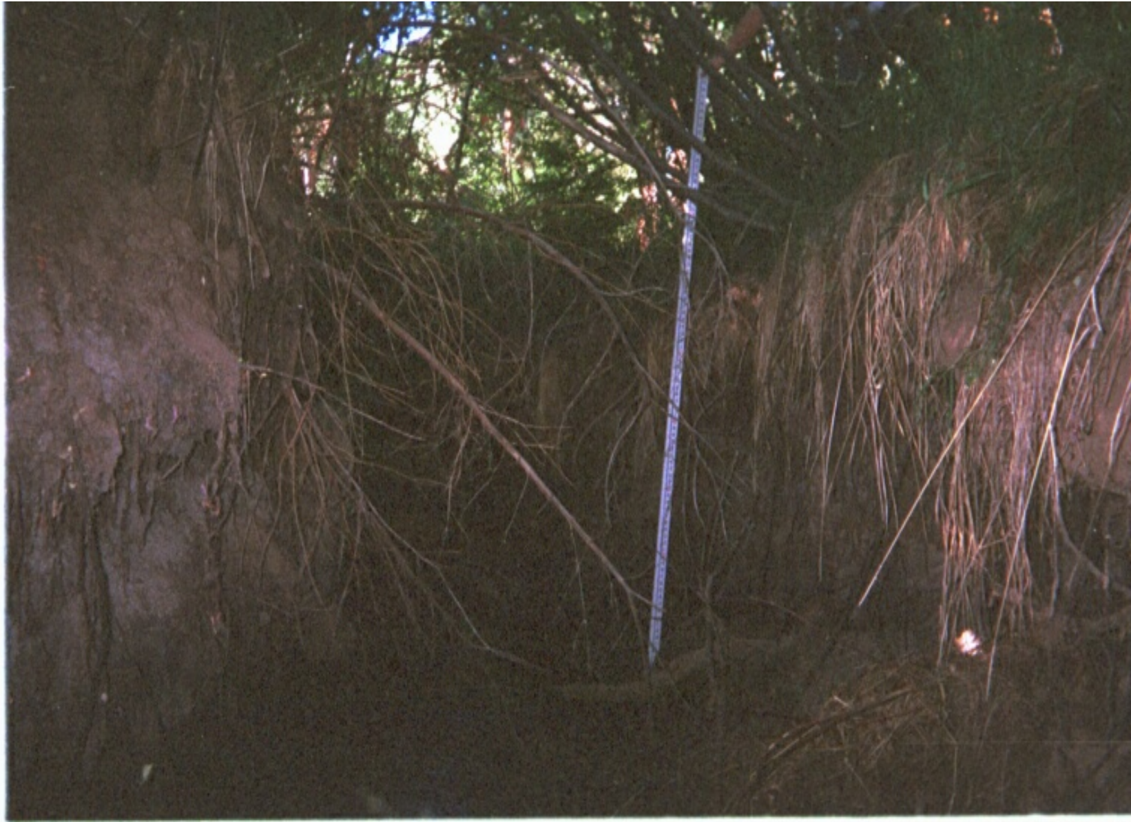
Figure 5-10. Channel incision and bank erosion on Rosewood Creek. The bank height is over 7 ft about station 52+40.
