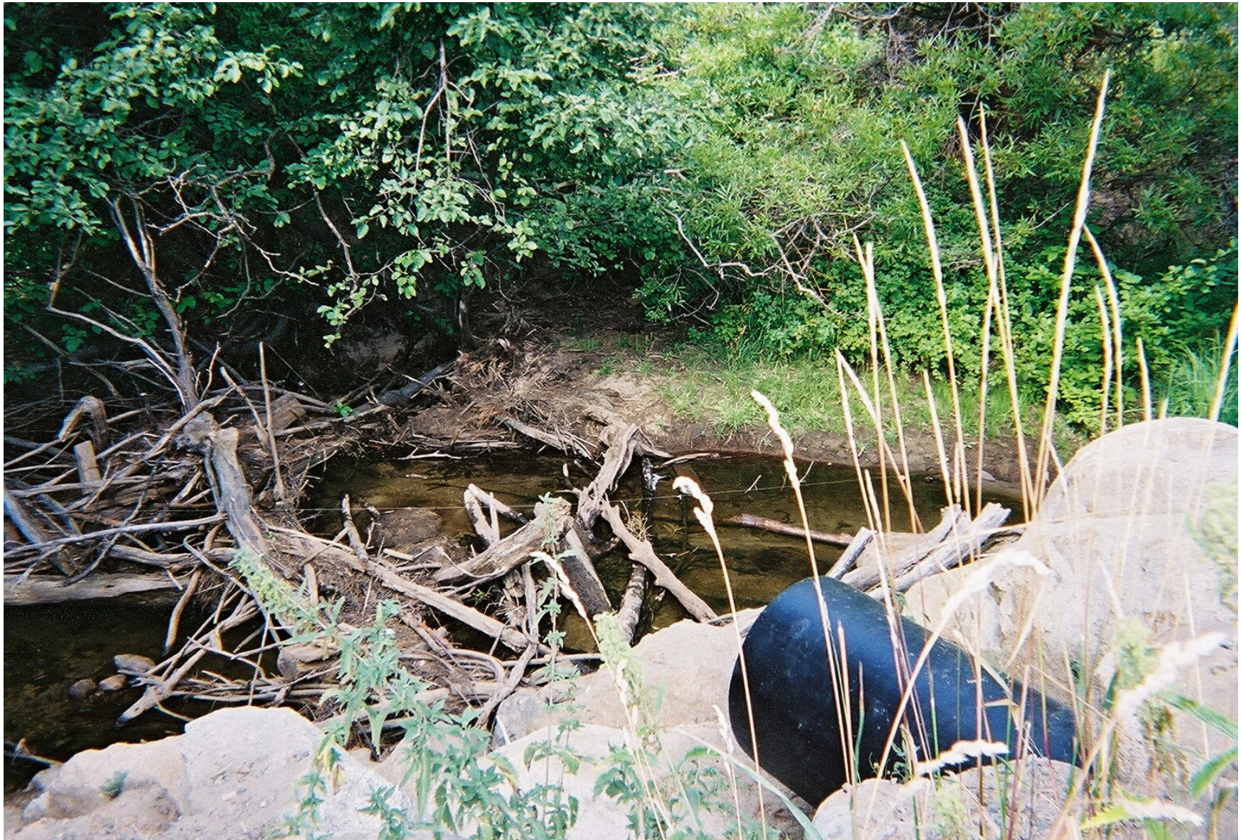
Figure 5-2. Photograph of sand impounded behind a woody debris jam on Third Creek. This site is located about 600 ft downstream of Incline Way near station 18+50.
