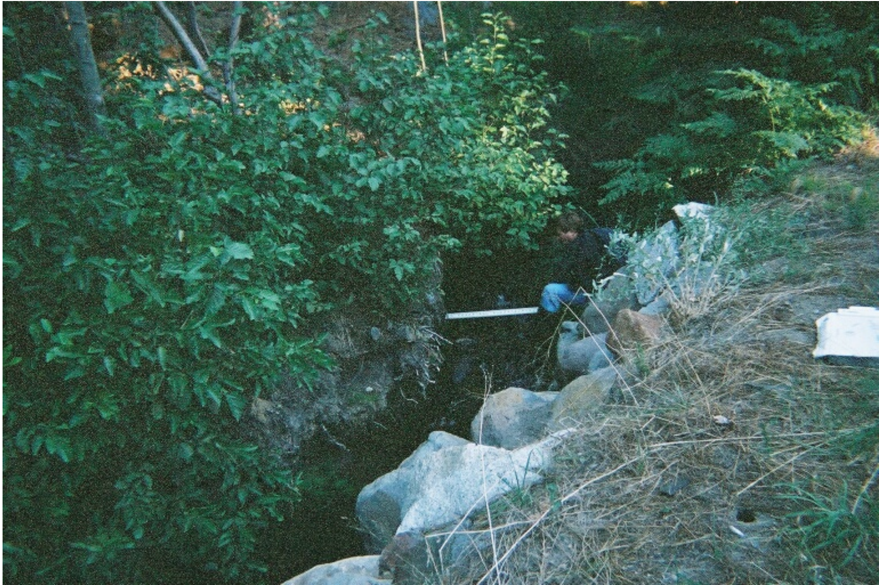
Figure 5-12. Undercut bank (approximately 1.5 ft) on Rosewood Creek along Village Blvd. Rip-Rap placement on left bank is likely accelerating erosion.
