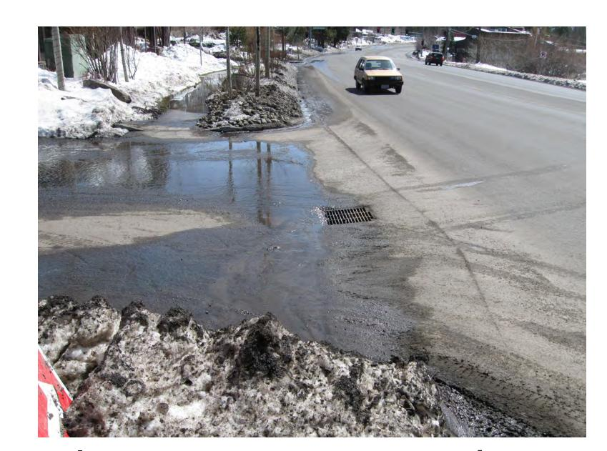
Drop inlet conveys untreated stormwater from Hwy 50 directly to Burke Creek.
