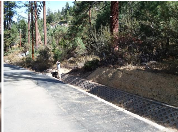
Rock lined channel with infiltrating drop structures and block channel leading to micro-basin.
