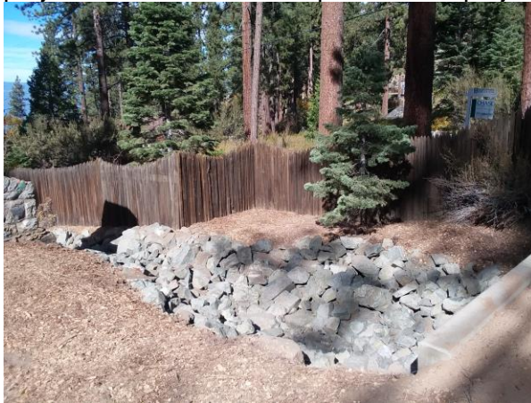
Rock lined channel with infiltrating drop structures and block channel leading to micro-basin.
