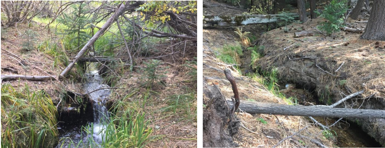
Figure 1. South Fork Marlette Creek has active down-cutting and remnant gabions from abandoned pipes.
