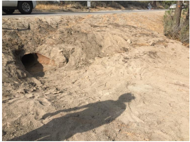
Figure 3. Stormwater pipes from State Route 28 discharging to Marlette Creek via untreated overland flow.
