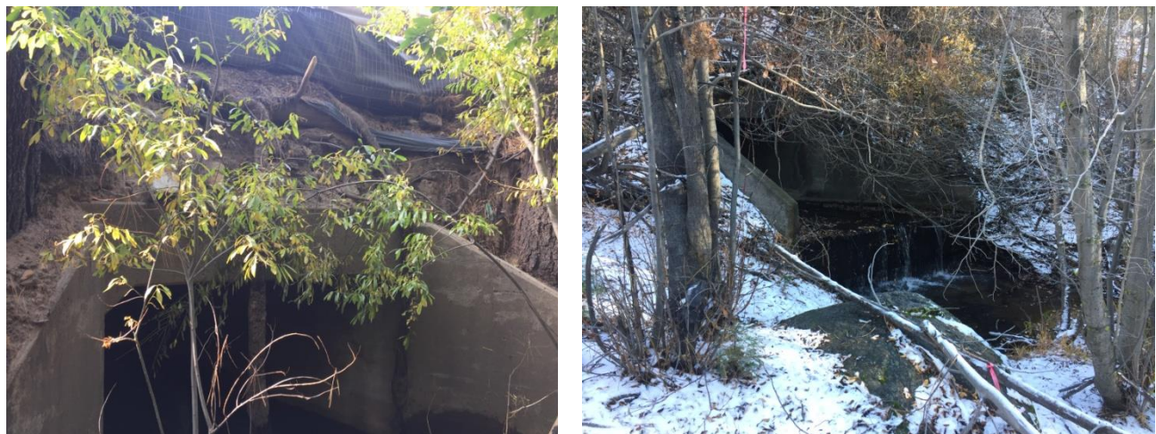
Figure 2. Left: Upstream end of culvert could be extended to reduce road embankment erosion. Right: downstream end of culvert has large drop measuring 3-4 feet.
