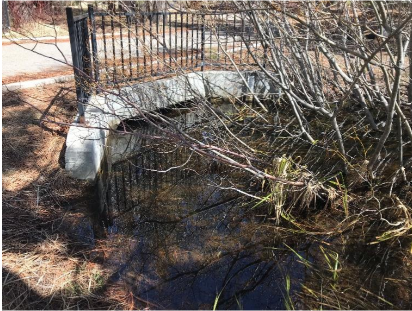
Figure 4: Concrete box culvert in Nevada Beach Campground at capacity during spring runoff, April 2019 (Photo: NTCD)
