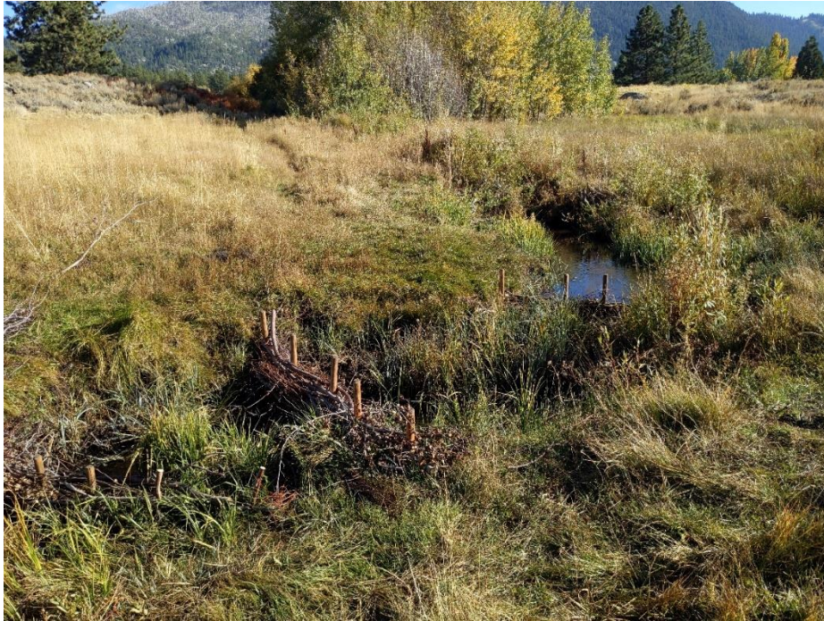
BDAs on Burke Creek shortly after installation in 2022
