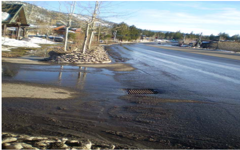
Photo 1.1. Directly Connected Drop Inlet to Burke Creek
