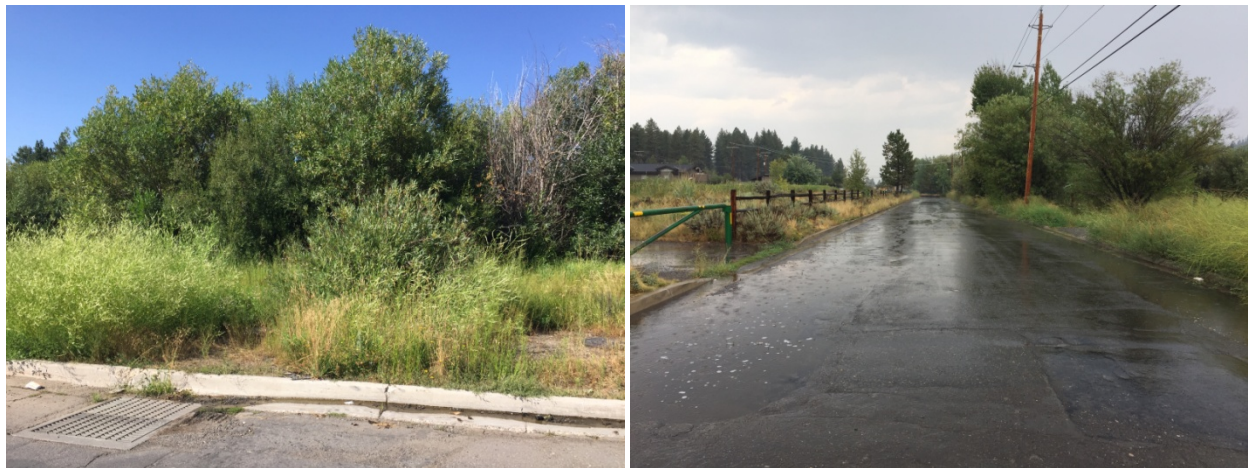
Figure 2. Left: Kahle Drive has undersized drainage that is constantly inundated with groundwater therefore stormwater cannot be captured and delivered to a treatment facility. Right: Kahle Basin is undersized and full of dense woody vegetation.
